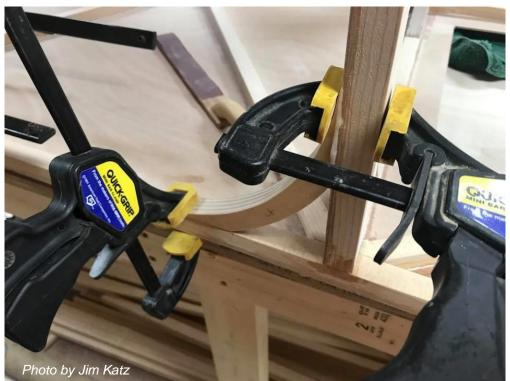
Figure 23: Gluing Corner Bows
