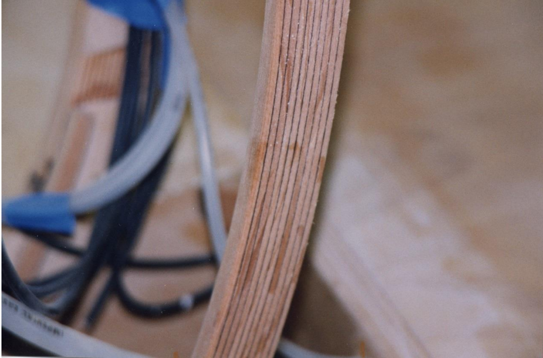
Figure 39: Close-Up of Lamination
