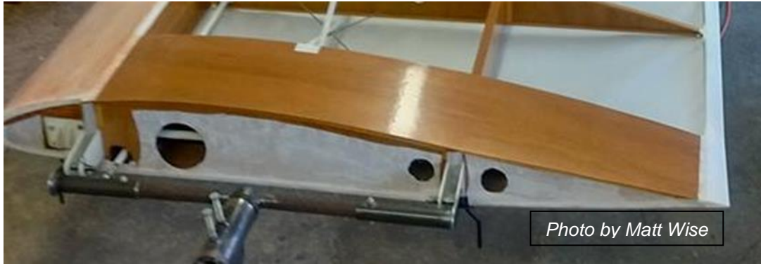
Figure 33: Access Holes Added to Rib 11
