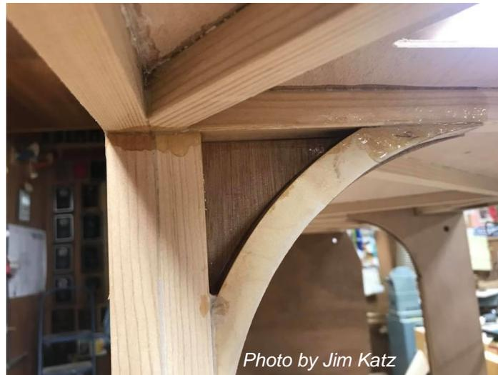
Figure 38: Varnish inside the Corner Bows
