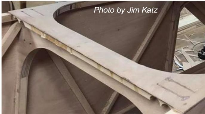
Figure 25: Slots for Landing Wire Anchors
