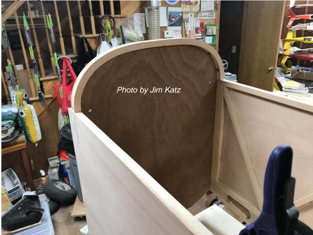
*Figure 9: Doubler on Top of Firewall*
