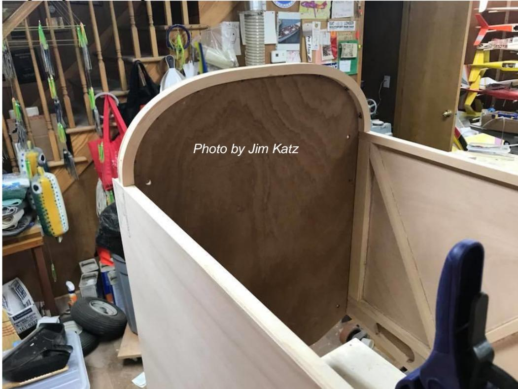
*Figure 9: Doubler on Top of Firewall*
