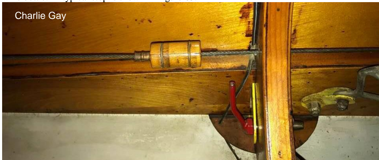
Figure 63: Stop Installed on Rudder Cable
